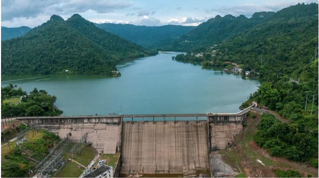
Figure 2 - Dos Bocas Hydroelectric Plant
